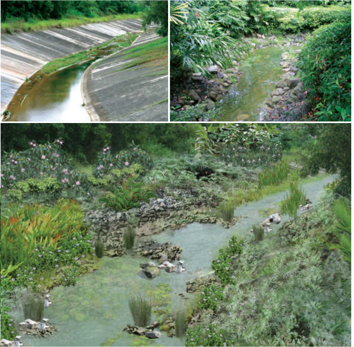
A concrete canal in Singapore (top left) can be “greened-up” to emulate a naturalised stream (top right). A wide selection of plants from different zonations can be selected to naturalise our existing concrete canals and also to lower the nutrient loads of the water in our waterways and waterbodies (bottom, Copyright: Touche Designs).
